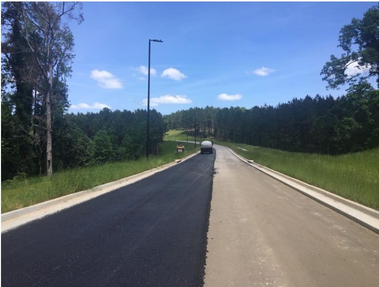
Construction continues on Hills & Dales Farm Road
