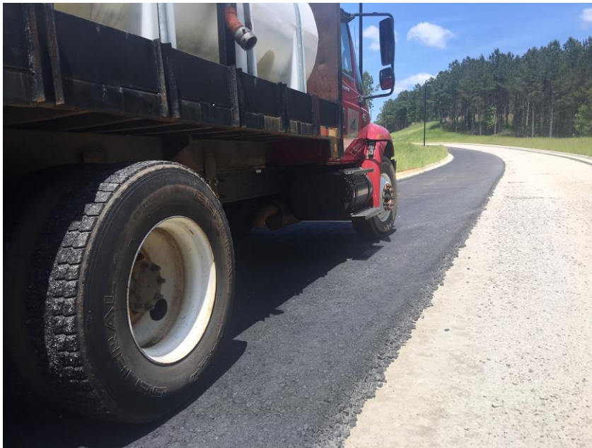
Construction continues on Hills & Dales Farm Road
