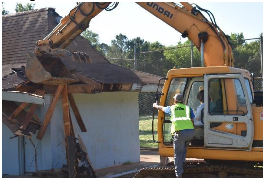
City Manager Meg Kelsey assists in the demolition
